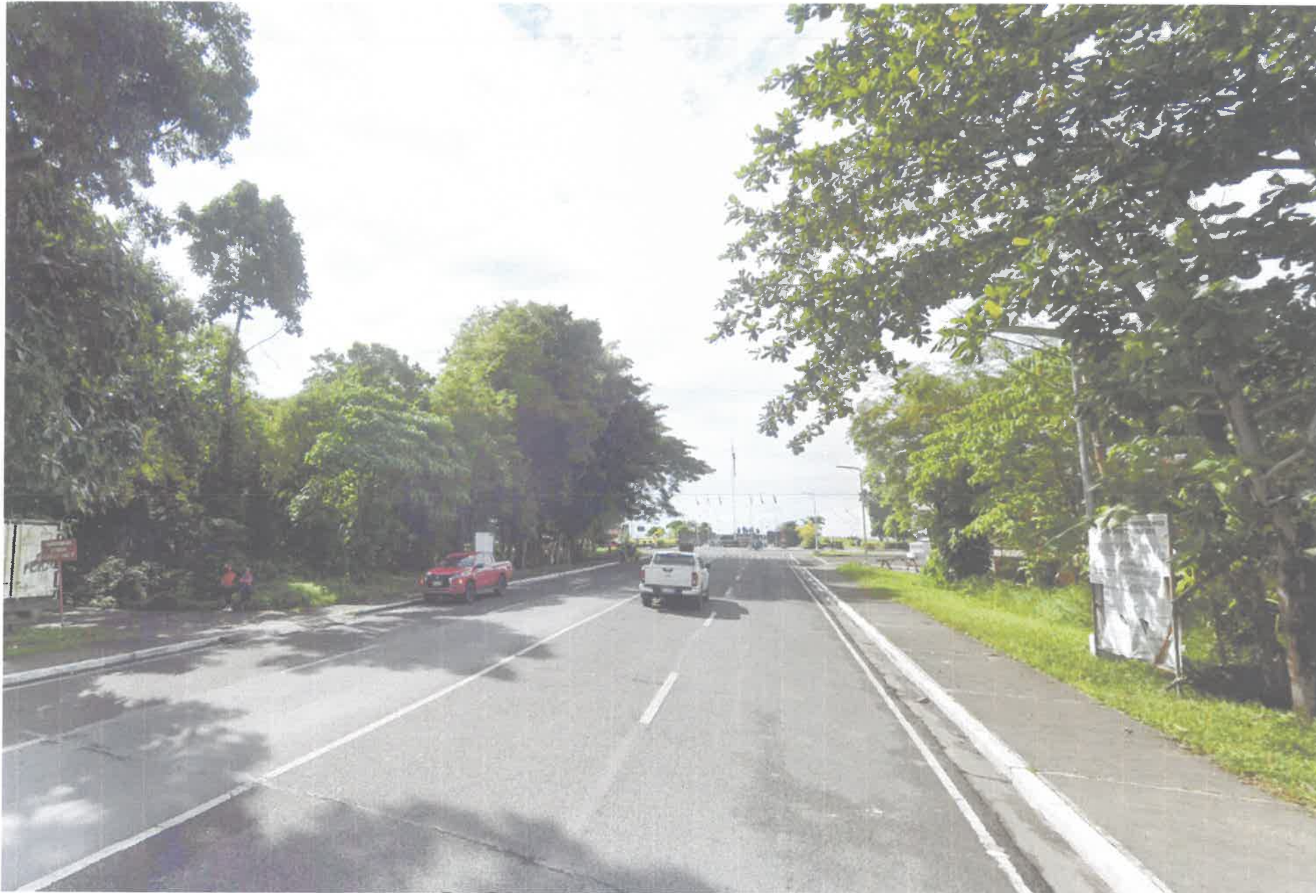
Existing Site Condition – Maharlika Highway MacArthur Landing Memorial National Park
