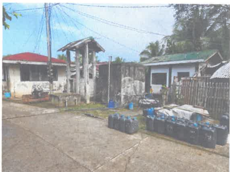
Concrete Reservoir at Naulayan Proper.
