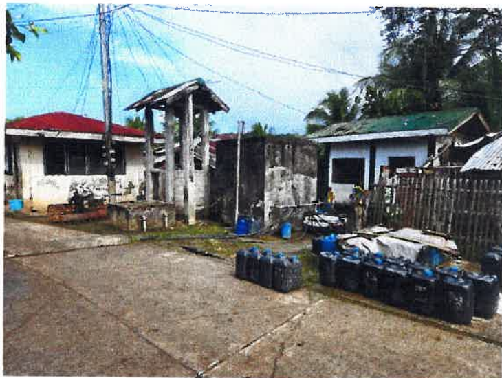
Concrete Reservoir at Naulayan Proper.
