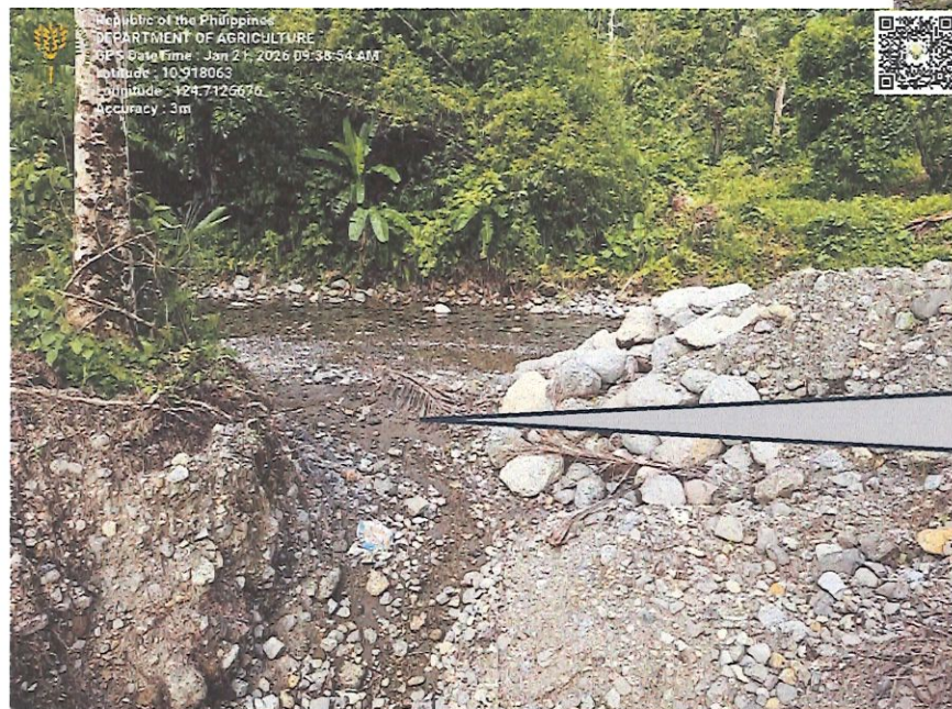
Picture showing excavation for settling pond outlet going to river
